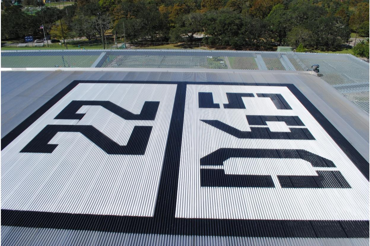
Picture 7. New Helistop enabling a larger aircraft with a maximum weight of 22,000 pounds and a rotor diameter of 65 feet. This is a benefit for natural disasters.
